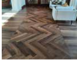
Polo Club, Emaar Installing parquet in different alignment
