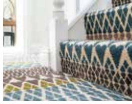
Private Villa, Abu Dhabi Installing carpet flooring
